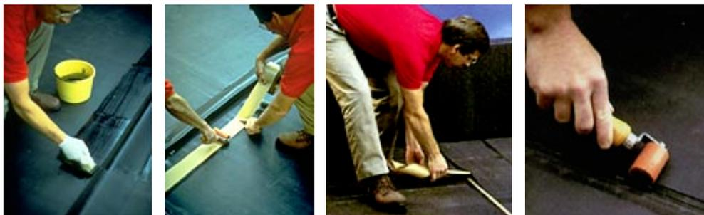
**Multiple Firestone EPDM Geomembrane panels can be assembled on site using the Firestone QuickSeam Splice Tape System. This advanced method of EPDM field seaming is based on Firestone QuickSeam Splice Tape, a self-adhesive EPDM/Butyl tape. Since its first application in 1987, millions of linear meters of Firestone QuickSeam Tape have been successfully installed worldwide.**
